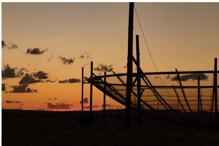
The HERA telescope array in South Africa. The array is a large grid of 14 meter (42 ft) diameter non-tracking dishes packed into a hexagonal grid 300 m (900ft) across. (Images courtesy of the HERA Collaboration.)
